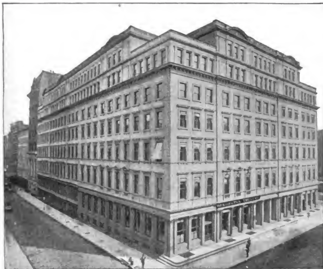
THE WASHINGTON TRUST COMPANY, STEWART BUILDING, 280 BROADWAY.
